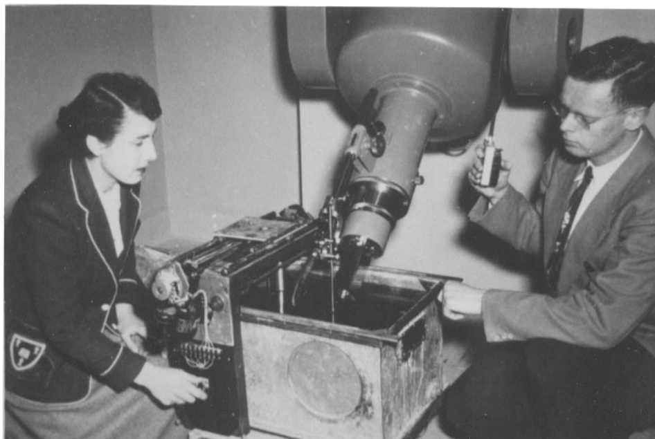
Sylvia Fedoruk and Ed Epp making isodose measurements for conical rotation therapy. Saskatoon, November 1951
