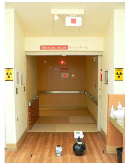
Figure 1: Status of the upper warning light above door is uncertain due to nearby skylight (source: CNSC file)
